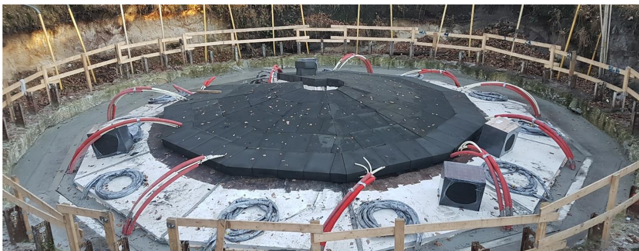
Centralized P2H solution in Uden (Netherlands). Large thermal storage facility to heat office and domestic buildings.
