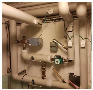
*Figure 2: Clamp-on temperature sensors at place in the second installation.*
