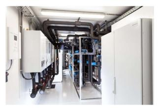
Figure 4: Pilot site in Uden, inside the technical room. From left to right: control unit for the AW heat pump; 6 boilers; WW heat pump; piping (black) and valves(blue); control cabinet.
