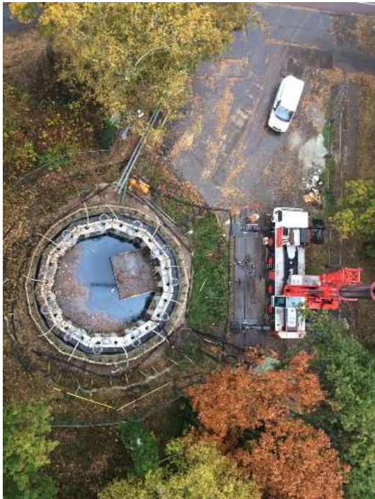
Figure 1: Ecovat pilot site during construction
