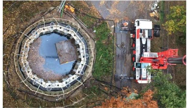
Figure 3: Ecovat vessel at the pilot site in Uden under construction.
