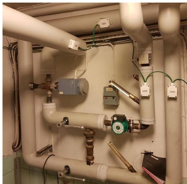
*Figure 2: Clamp-on temperature sensors at place in the second installation.*
